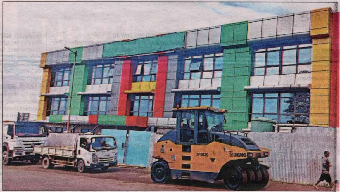
The complex to house the Eastern Highlands education division. PICTURE: SUPPLIED
